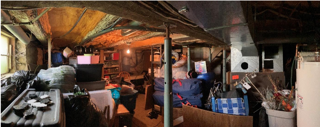
Plate 25: View of basement from southeast corner
