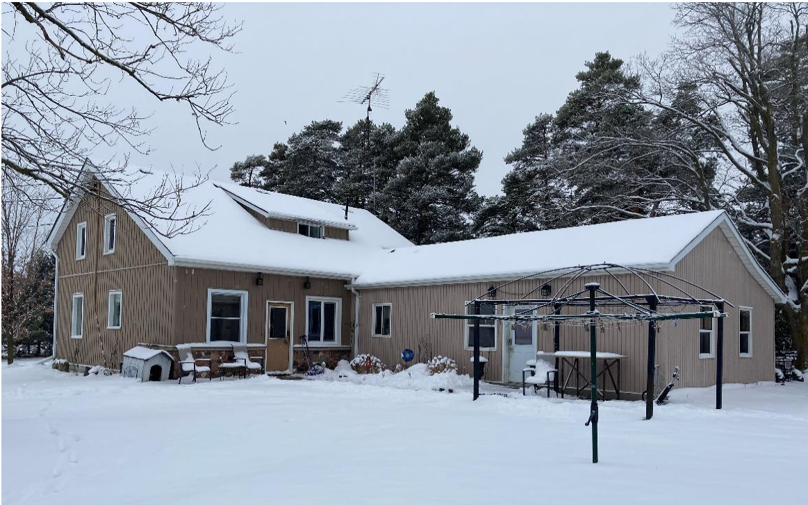
Plate 12: Oblique view of south and east elevations
