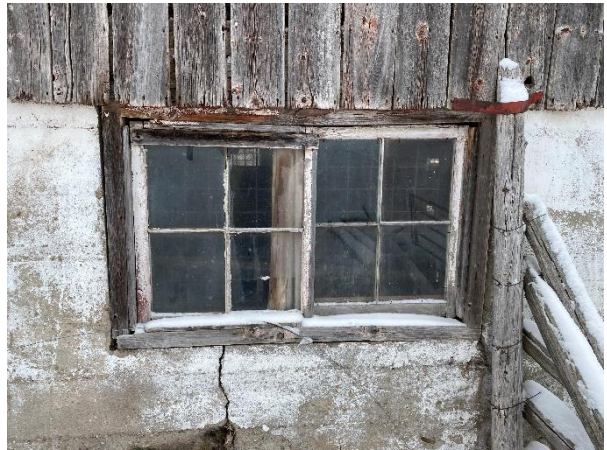
Plate 62: Barn No. 2 window detail.
