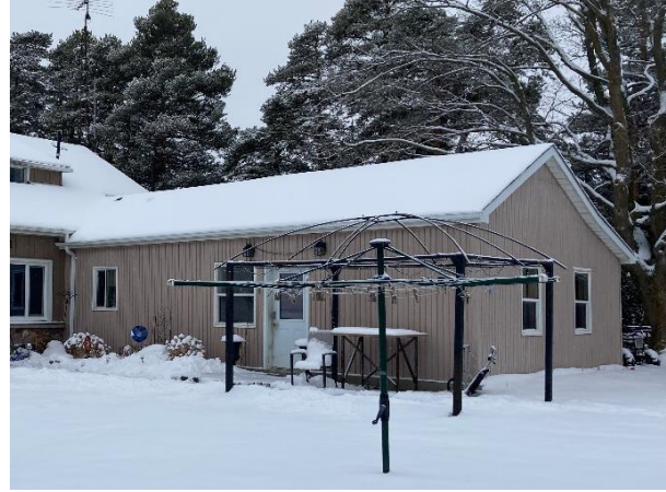
Plate 54: South and east elevations.
