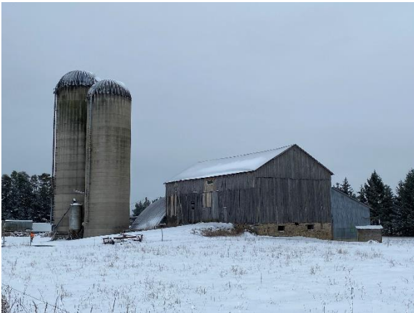
Plate 57: North and west elevation of Barn No. 1.
