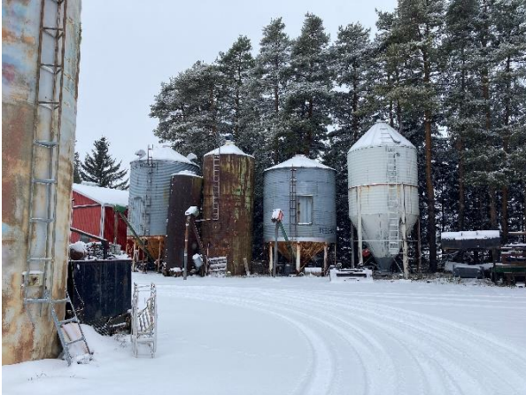
Plate 71: Additional silos between Outbuildings No. 3 and 4.
