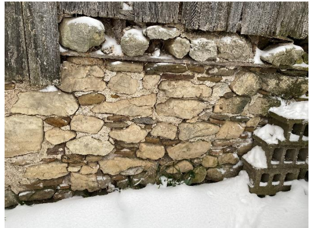
Plate 58: Detail of Barn No. 1 fieldstone foundations.
