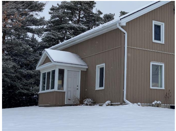
Plate 22: West elevation enclosed porch.
