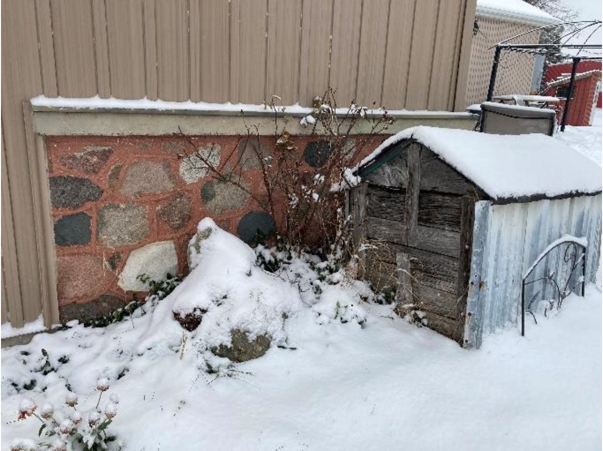
Plate 52: Fieldstone veneer indicating the limit of porch addition on main block.
