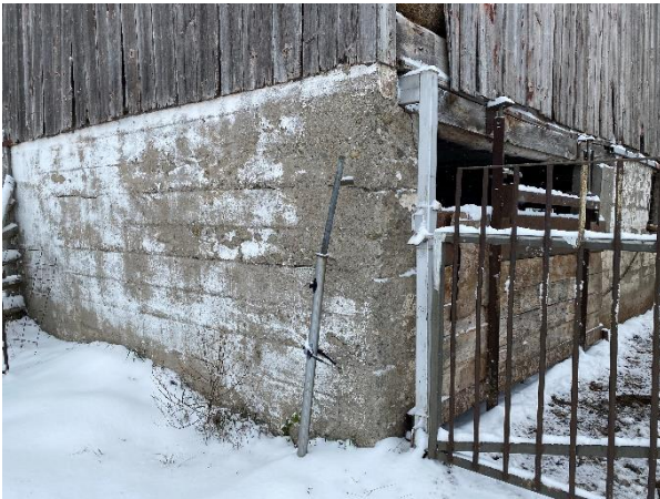
Plate 61: Concrete foundation of Barn No. 2.
