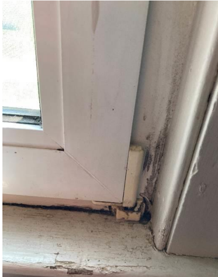
Plate 49: Second storey window
