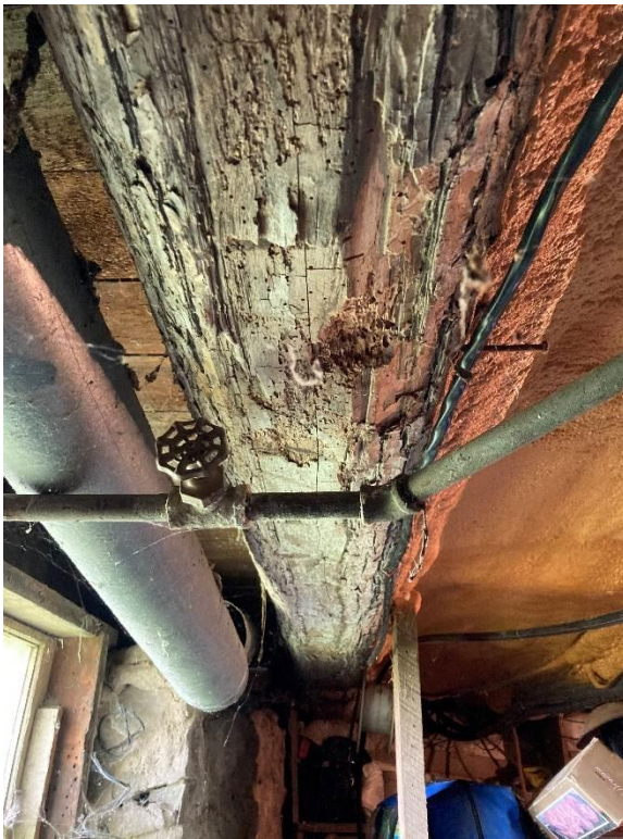
Plate 29: Hand hewn timber floor joist
