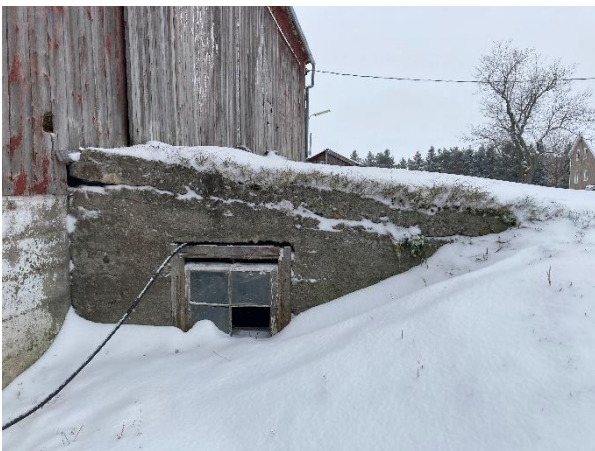
Plate 63: Barn No. 2 wingwall window.
