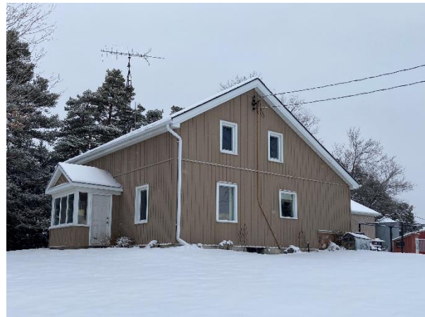
Plate 18: Oblique view of south and west elevations
