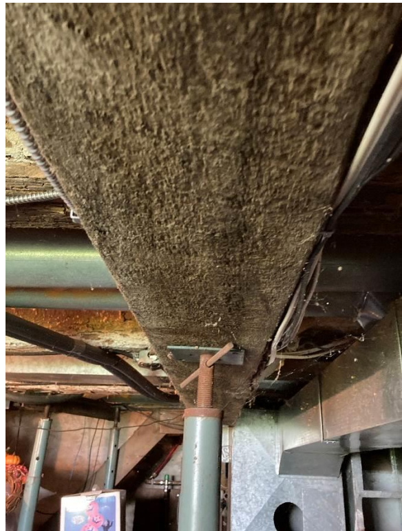
Plate 30: Machine cut timber floor joist
