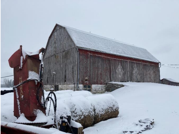
Plate 59: North and west elevation of Barn No. 2.
