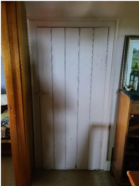
Plate 47: Original wood plank closet door
